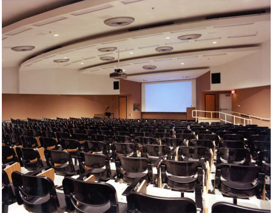
The three-level light system, comprised of cove lights, recessed fluorescents, and recessed cans, gives the room a different ambience according to the instructor's needs and wishes.
