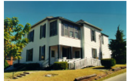
The existing structure.
