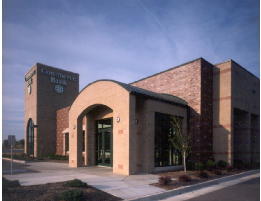
The prominent sign tower catches the attention of all who pass by this building.
