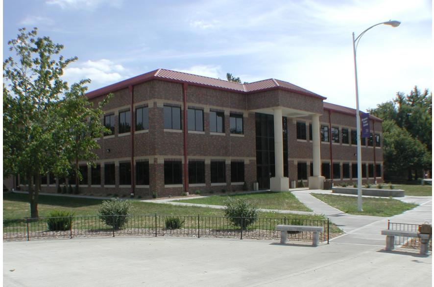
The Technological Library/classroom addition is serviced by fiber optics and accomodates 65 work/computer stations.
