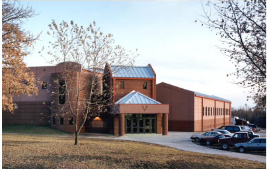
The structure of pre-cast stone walls and colored metal roof is a striking addition to this campus.
