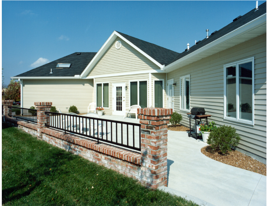
The back of the Machens home is completely wheelchair accessible.
