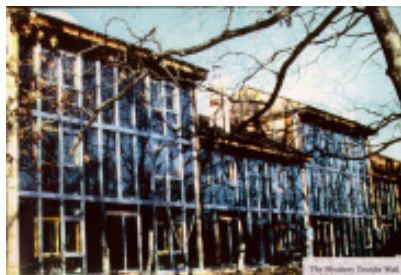
The Trombe Wall townhomes.
