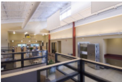
Light-colored materials, banners and a light shelf help to illuminate the interior of the building.
