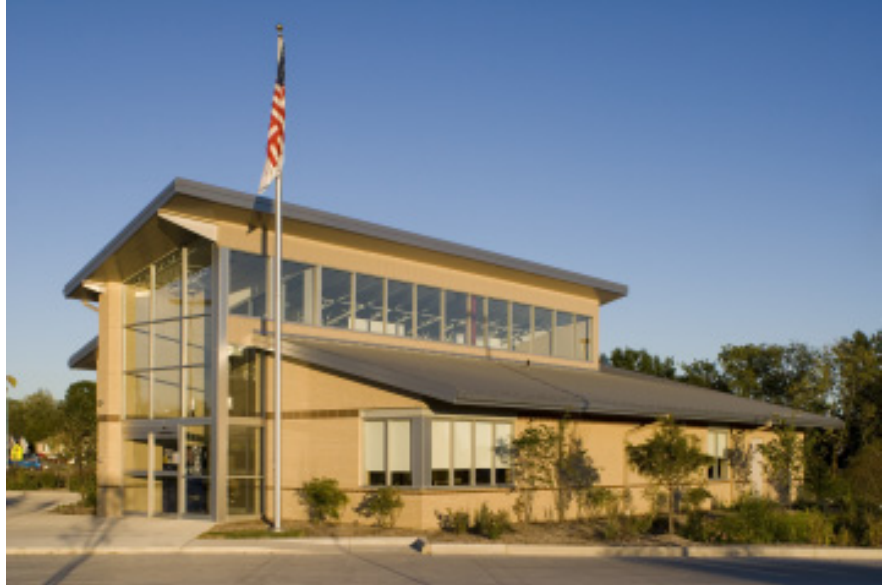
Clerestory windows on the south side of the building bring indirect natural light to the interior spaces of the building.
