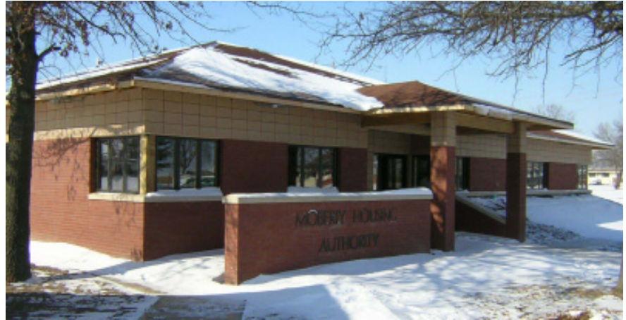
The recently dedicated Moberly Housing Authority Community Center includes many sustainable design practices.
