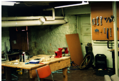
The basement storage room was dark and damp before it was renovated into a classroom.
