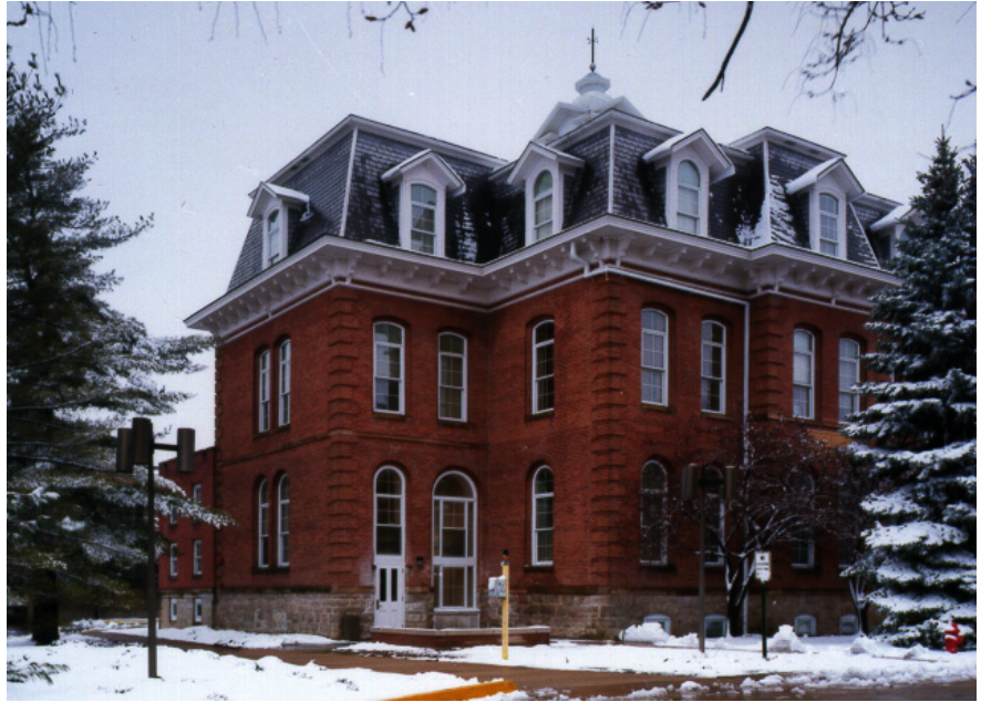
The front entrance was lowered to provide easy access. Photographs by Deanna Dikeman
