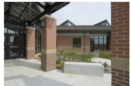
Clerestory windows have been used to let natural daylight deep into the interior space of the building.
